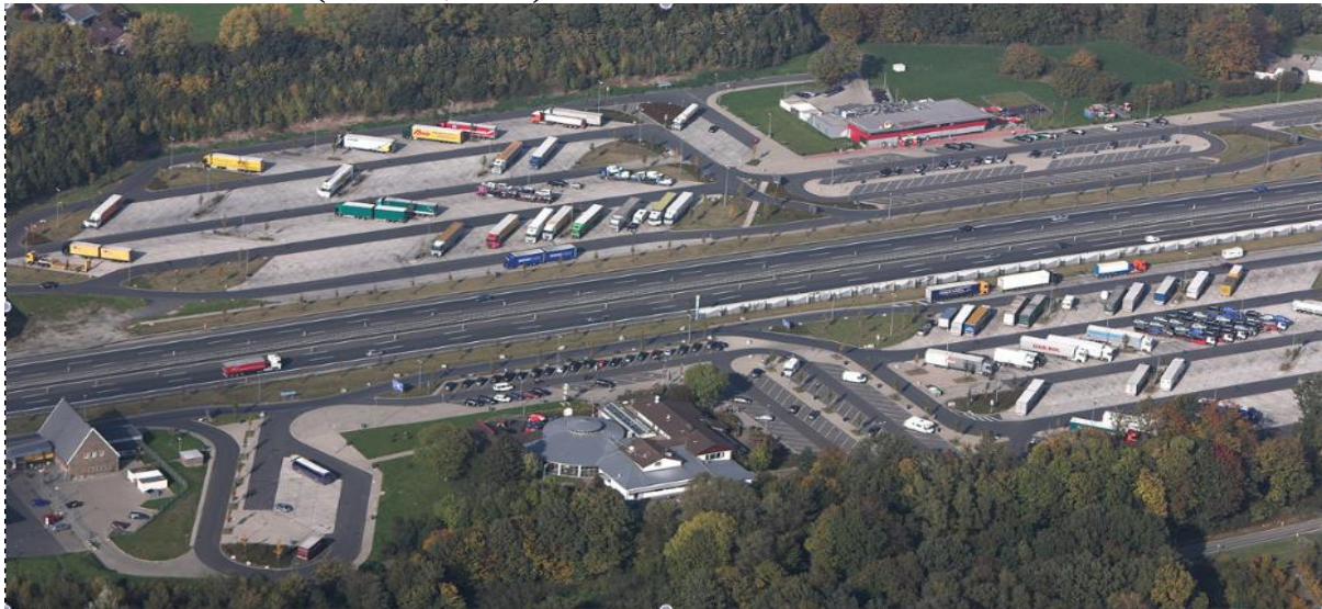
Plate 3: Izuwa (Modern TTP Facility). From Infrastructure Concession Regulatory Commission, Nigeria (2018).
